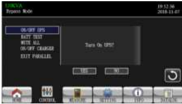
TURN ON UPS
