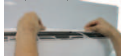
Figure 105: Disassembling the Air Filter (Appearances Will Vary Depending on Indoor Unit Model).
