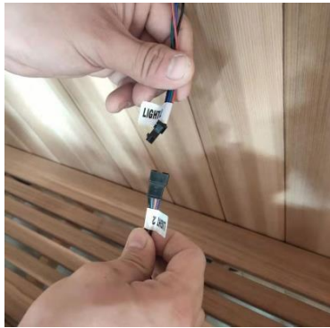
Rear Wall – Middle Light Connection
