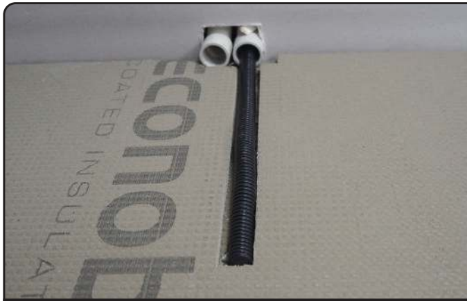
Push the supplied flexible conduit out into the channel in the floor. Ensure that the black cap is firmly in the conduit.
